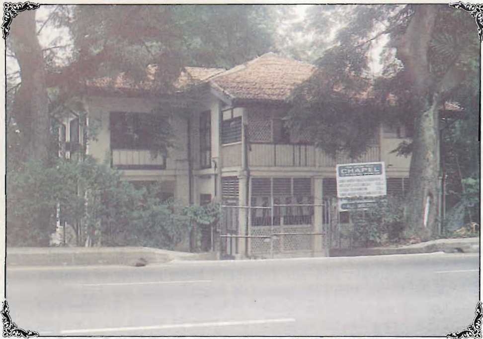
NEW BRIDGE ROAD CHAPEL LOCATED AT 417 NEW BRIDGE ROAD.
