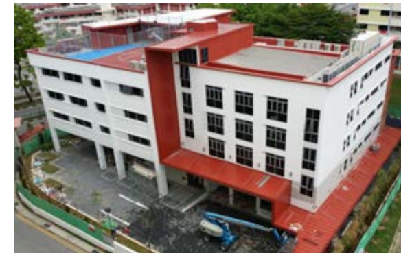
North-West aerial view showing the finished roof and rear canopy extended to the boundary edge. The red roof is designed to 'wrap around' the building, binding the old and new into one; just as the Old and New Testament form one complete Word of God.
