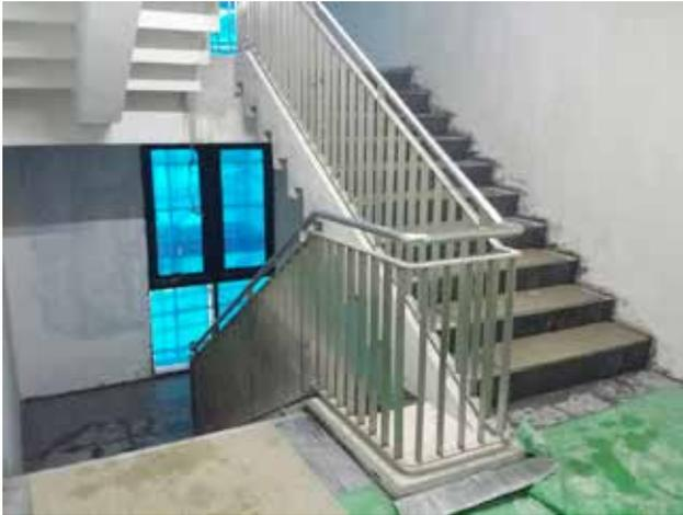
*All staircases are being retiled, and railings changed to high-grade stainless steel finish. This provides for better safety, better resistance to corrosion and hence requires less maintenance.*
