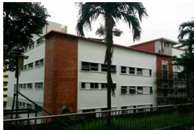
*View of the almost completed south façade seen from HDB Block 173. The red-brick vertical wall is the only externally visible remnant from the existing building. This is a deliberate attempt to preserve parts of the existing building, since this red-brick corner is significantly 'iconic'.*
