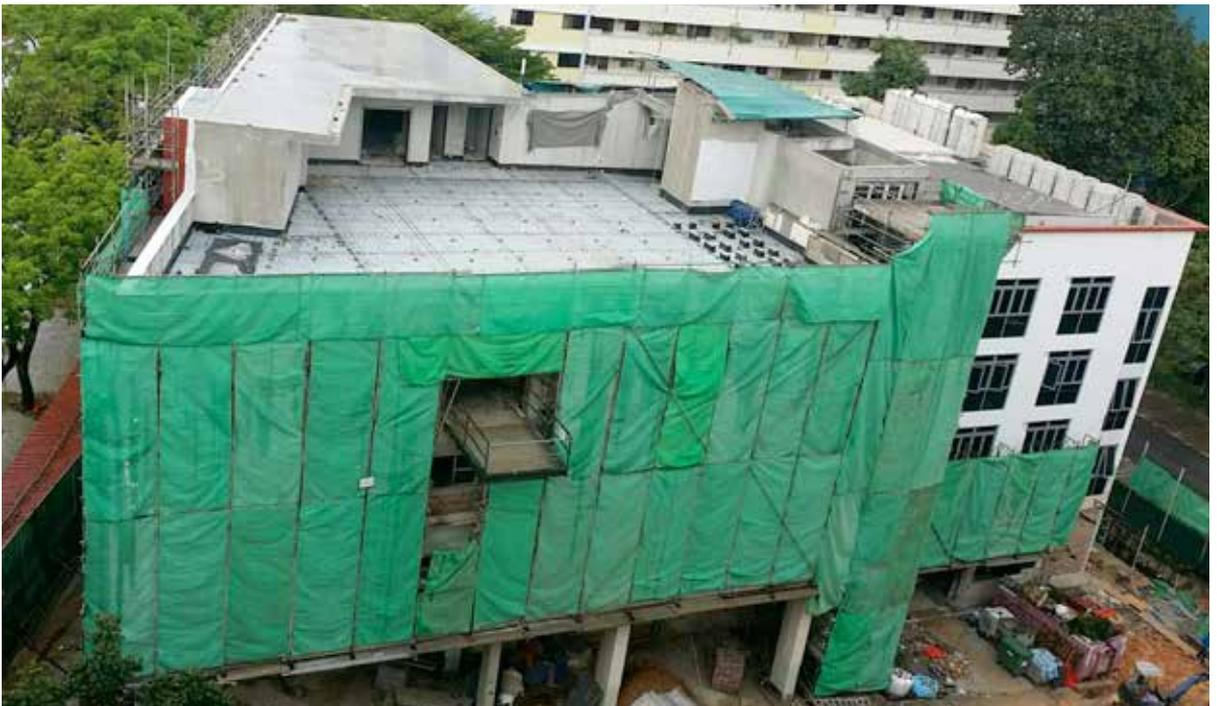
*Aerial view showing the completed 5th Storey awaiting the final layer of roof insulation and the finishing coat for the basketball court. The new rooftop function room is also completed. To the right, the front façade is slowly being revealed with the environmental netting progressively taken down.*
